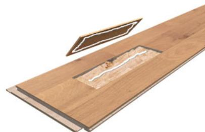
Select and fit a replacement strip. Fill the cavity with epoxy and press the strip down.
